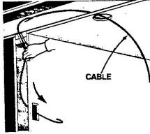
Attach the cable to the ceiling tape this time and pull it through the top plate to the cutout, and from there to the box hole.
